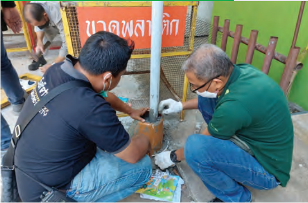
Improvement of Waste Sorting Plant
